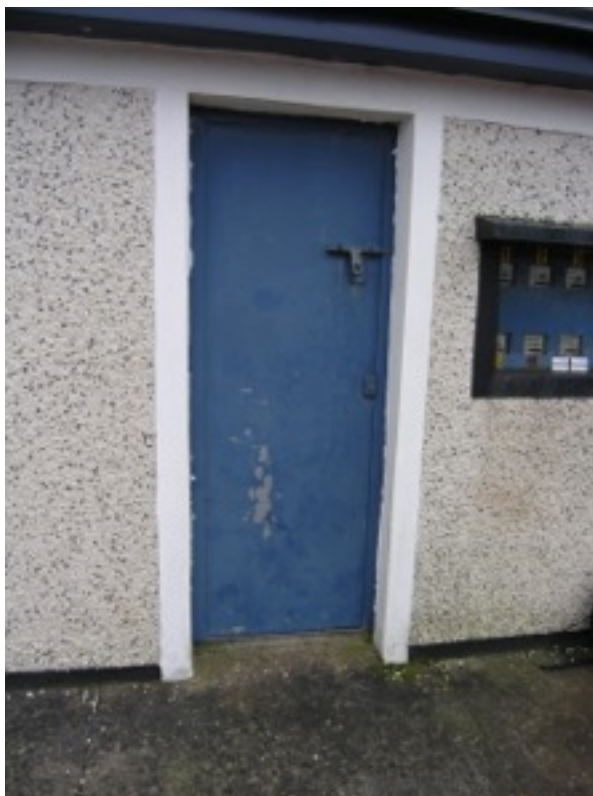
Left: Secure area, with meter boxes to right
