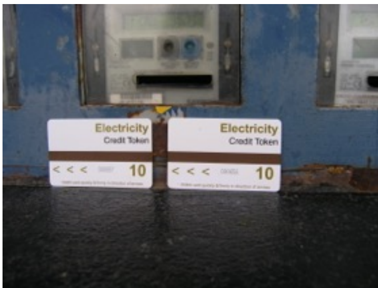
Left: pre-payments cards, with meter box in background.
